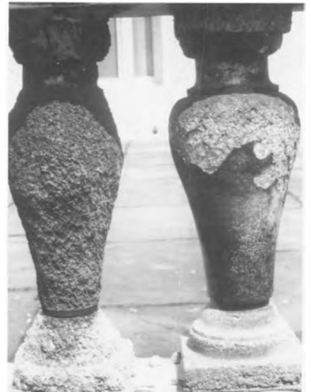
Fig. 5. Two marbles show significant differences in their resistance to weathering. The capital is Carrara marble; the shaft is Pennsylvania marble. This column is located on the south side of the east facade of the Merchants' Exchange, Philadelphia, Pa.
