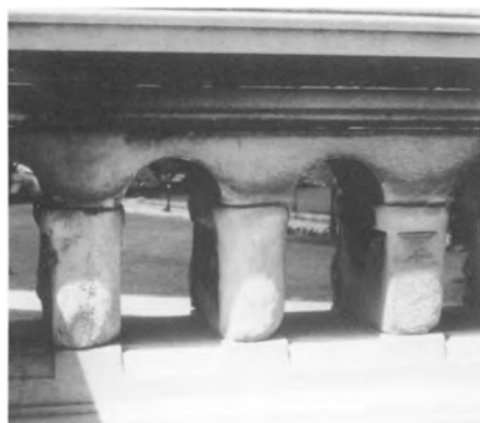
Fig. 1. Rounded edges are left by dissolution. Balustrade, U.S. Capitol, Washington, D.C
