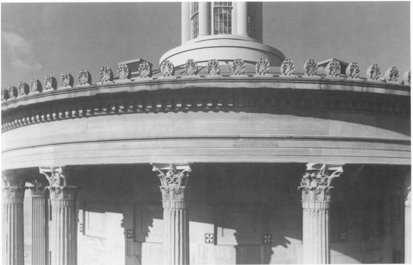
Fig. 10. East facade columns, Merchants' Exchange, Philadelphia, Pa.
